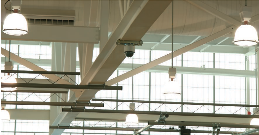
Three stories up, an Axis 233D camera monitors the main gymnasium and running track inside Adelphi's new sports center.
